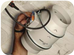
Carry out the wiring connections
