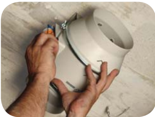
Place the impeller and motor
