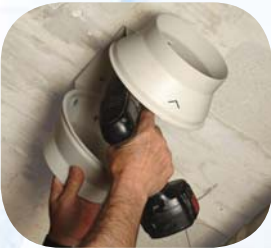
Fix the support bracket
