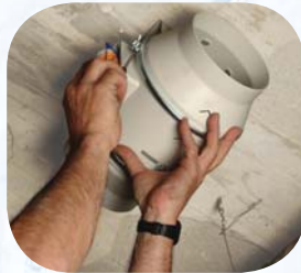
Place the impeller and motor assembly
