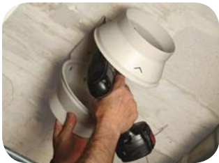
Fix the support bracket
