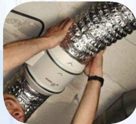
Connect the ducts
