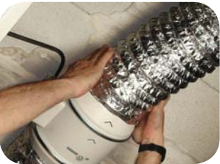
Connect the ducts
