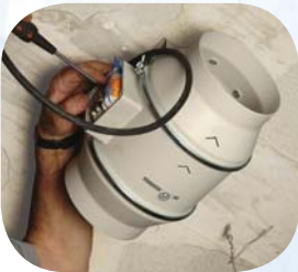
Carry out the wiring connections
